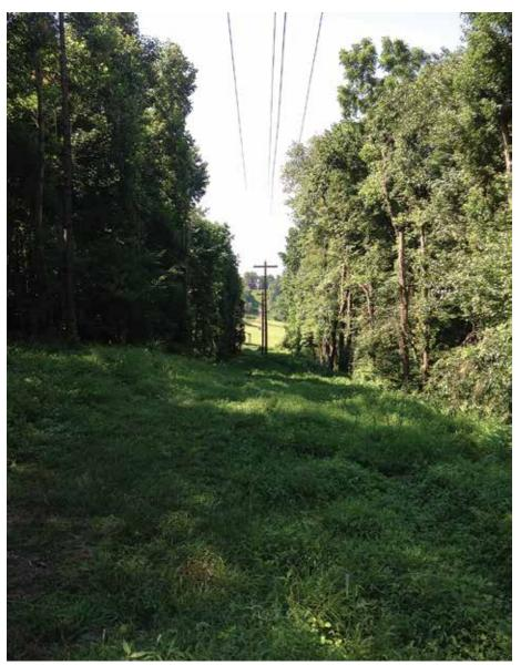
CLEAR VIEW: Following maintenance of a right of way near the Hanover Substation, members can now see a clearing where the co-op's power lines can run uninhibited, with less chance of tree damage or interference.
