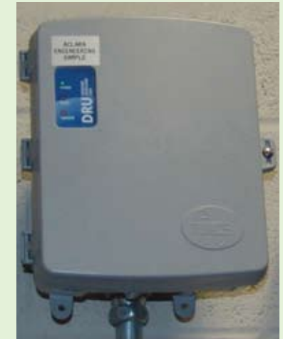
ADAMS ELECTRIC CONTINUES TO REPLACE ITS OLD LOAD CONTROL SWITCHES WITH THIS NEW VERSION.
